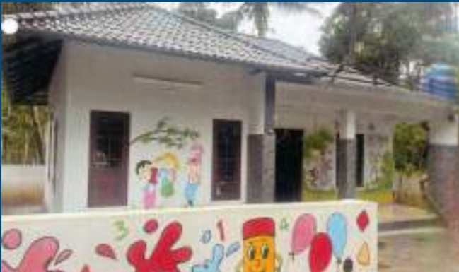
Construction of Schools at Wayanad, Kerala
